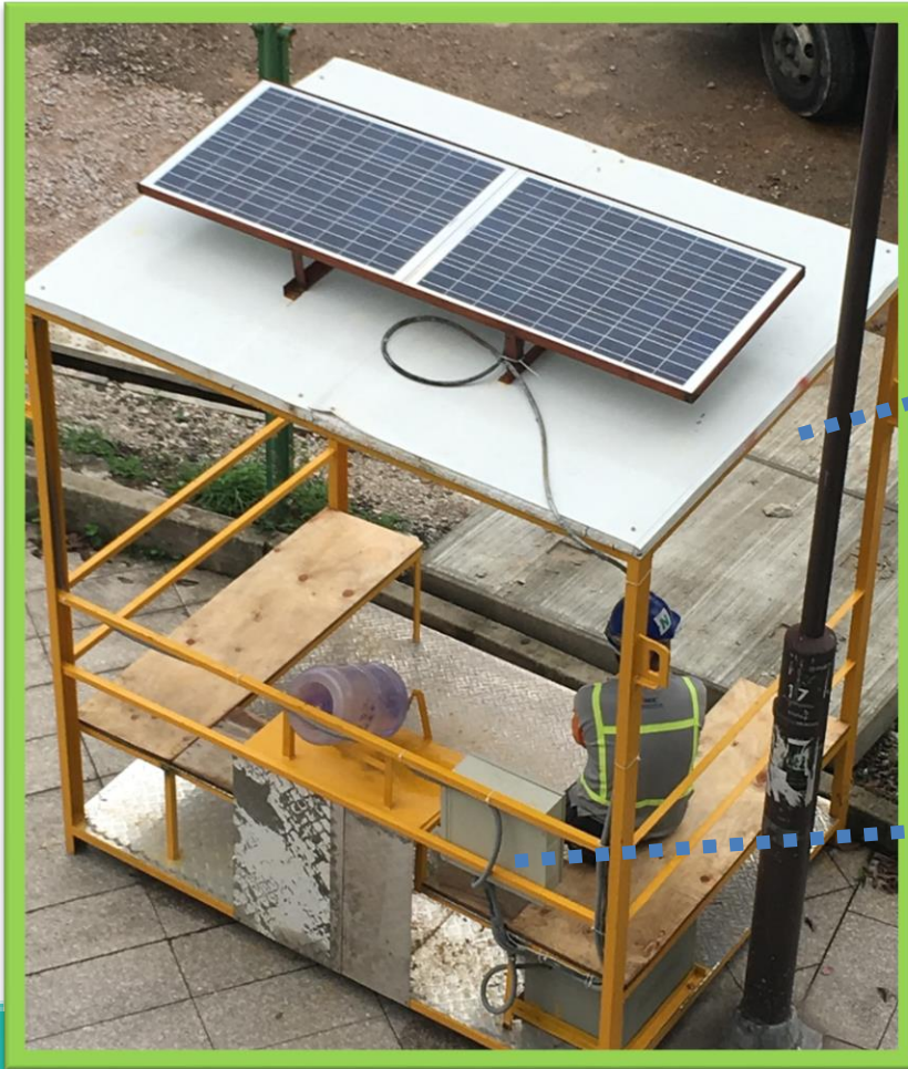
Solar energy for moveable workers rest area
