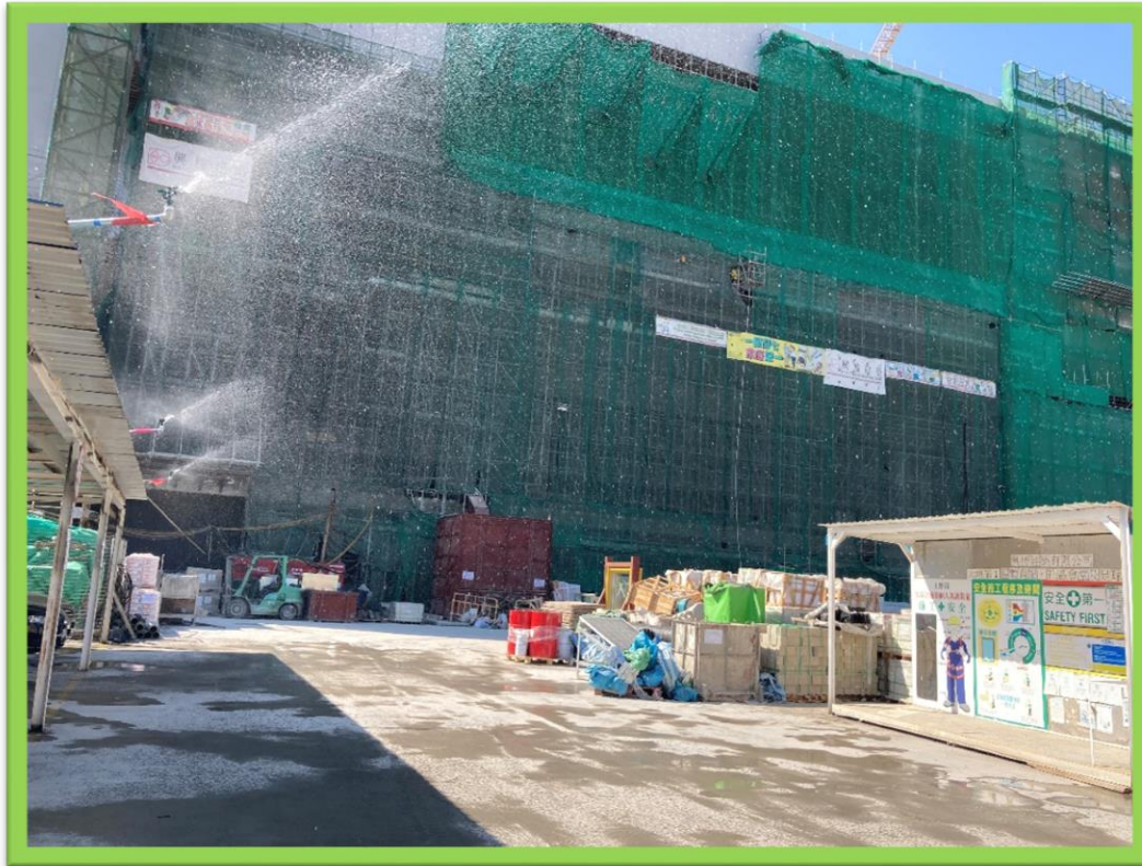
Water Spraying System for dust suppression
