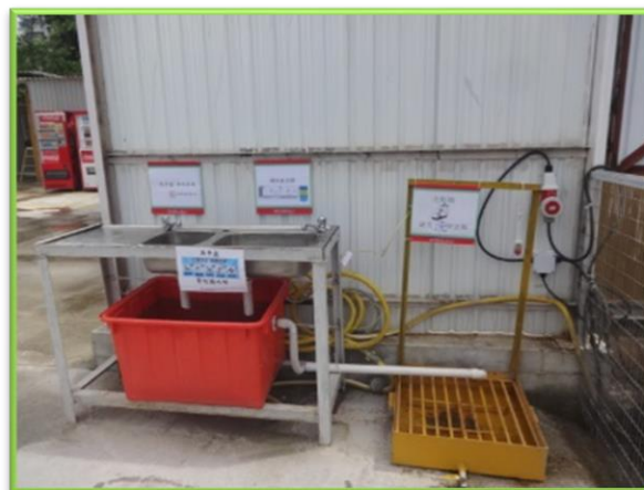
Using recycle water for shoes cleaning bath
