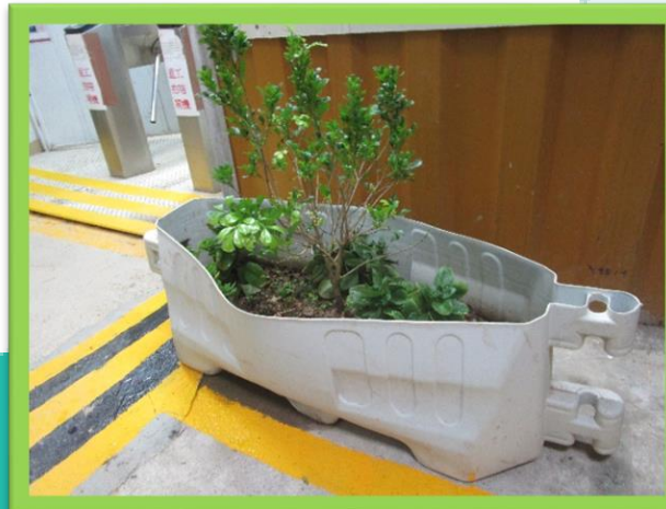
Recycle of Temporary Fence
