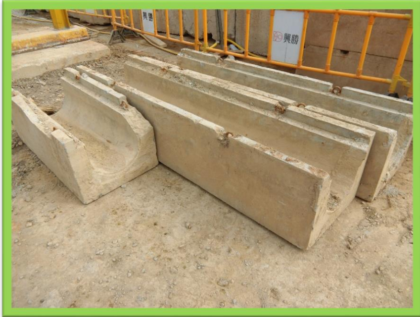
Pre-cast UU channel to reduce wastage
